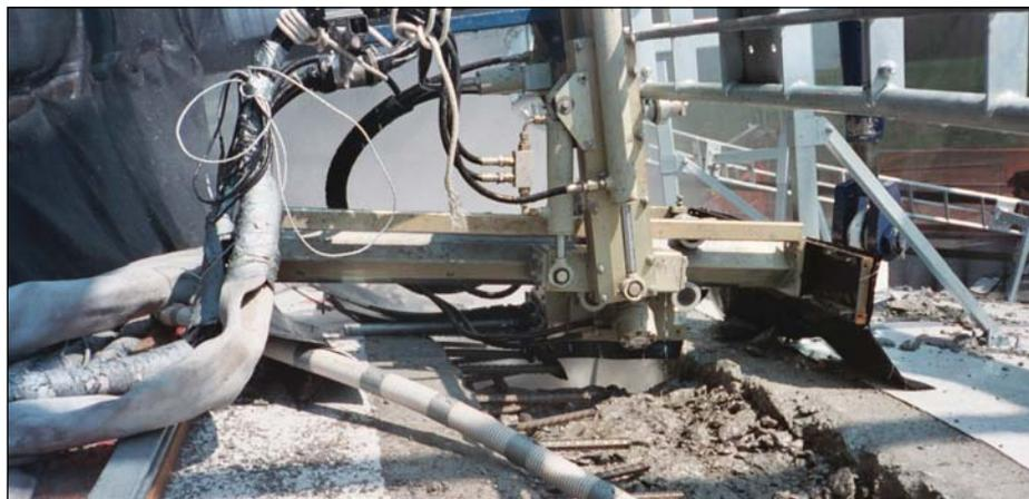
A robot, resembling a small bulldozer, has a camera mounted to its oscillating nozzle so operators can monitor the cleaning process.
