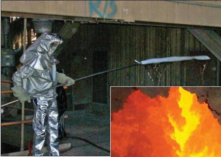
Blasters use telescoping poles to set the charge, which knocks slag off boilers and their tubes so Hi-Vacs or Guzzlers, pulling 27 inches of vacuum at 5,000 cfm, can vacuum it up.
